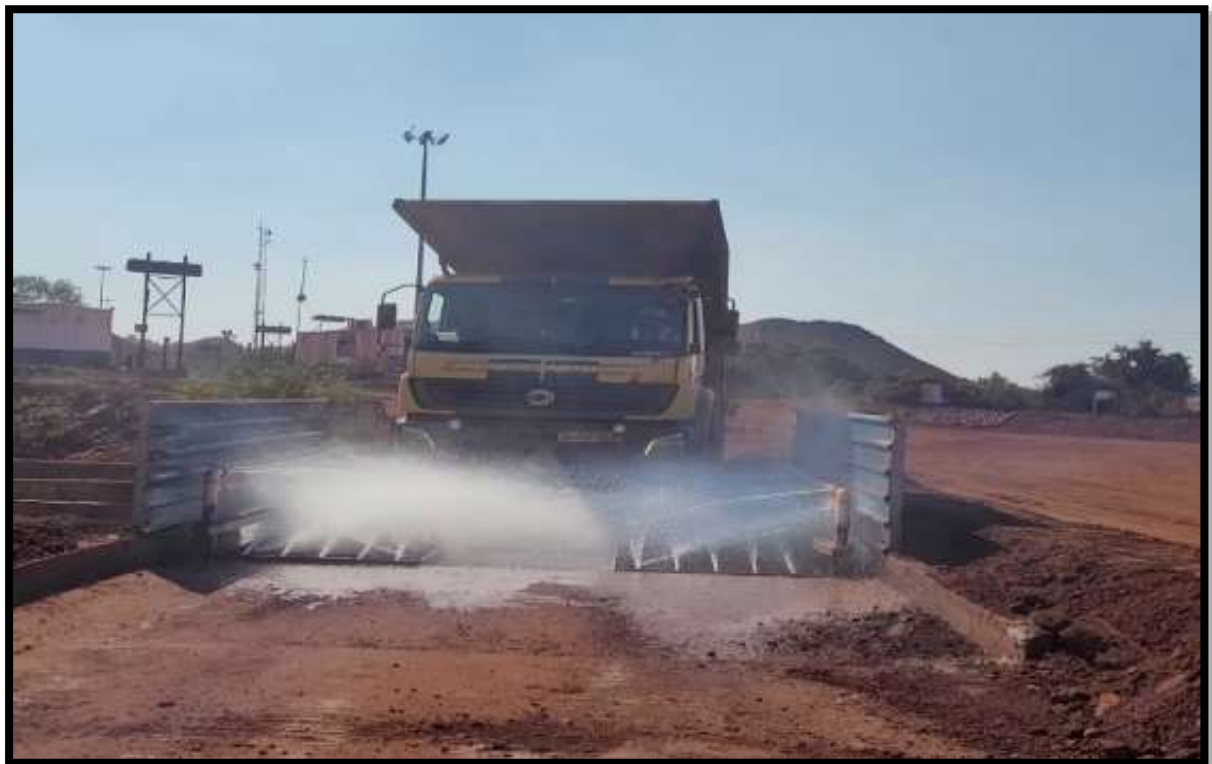
WHEEL WASHING POINT NEAR THE EXIT GATE
