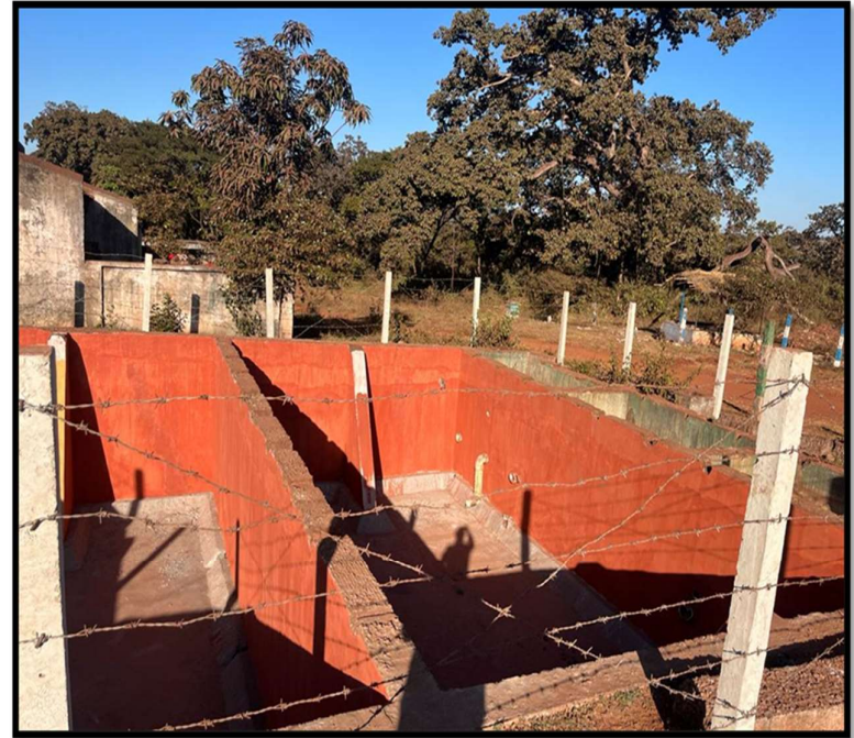
Collection pit of Rooftop Rain water harvesting
