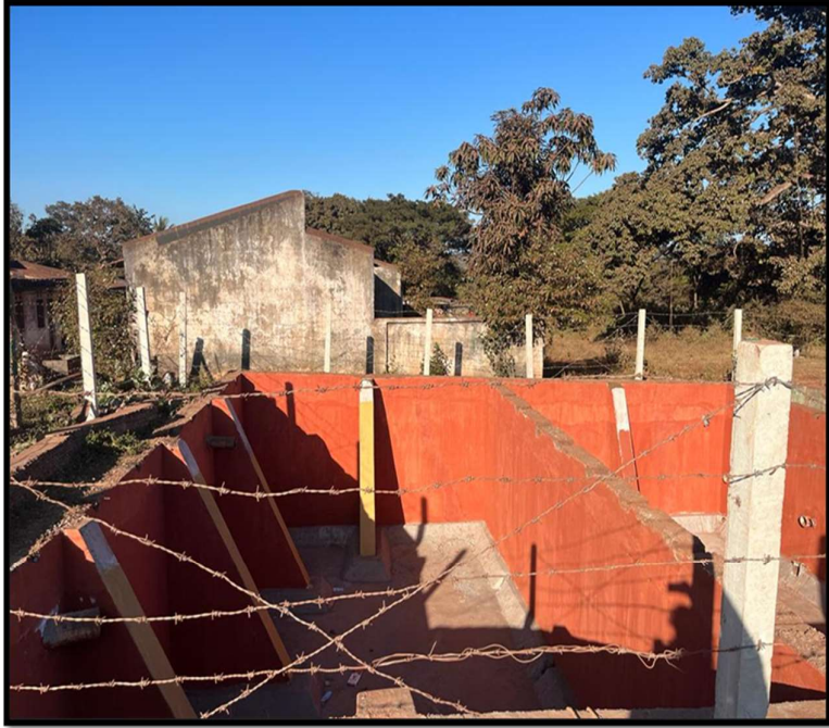
Collection pit of Rooftop Rain water harvesting
