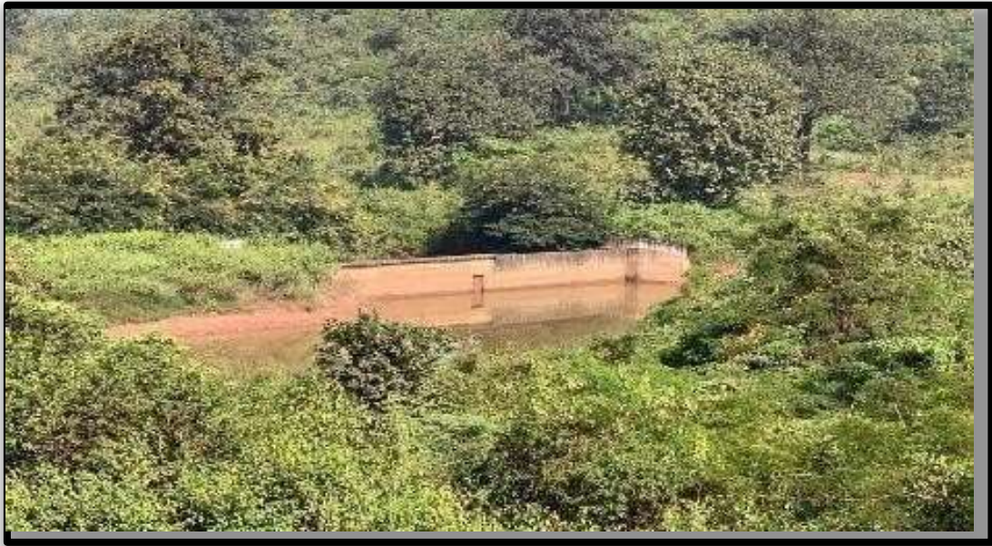
CHECK DAM, 40000 cum CAPACITY
