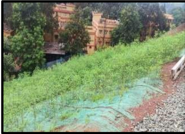
Retaining Wall, Geo Coir Matting & Plantation on Backfilled Area 2
